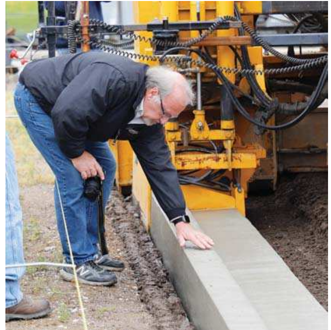
Picture 2: Dr. Mike Ayers inspects concrete curb and gutter with the MCE™ admixture
