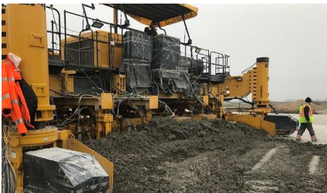
Picture 1: Concrete with MCE™ can be placed using traditional methods, including slipform paving.
